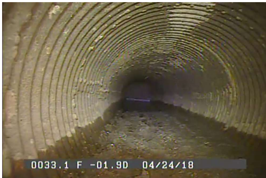
Needs to be Cleaned
